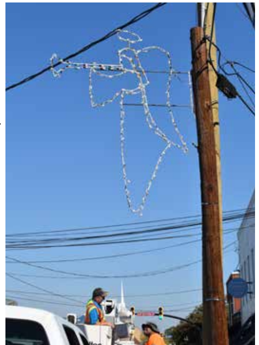
The Streets & Sewer Division of the Simpsonville Public Works Department installs 93 Christmas decorations over three days.
