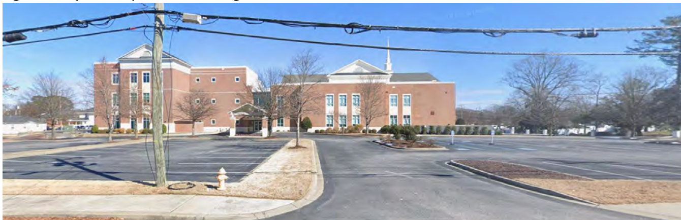
Figure 28: Upstate Baptist Main Parking Lot
